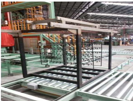
Treatment Process Systems
